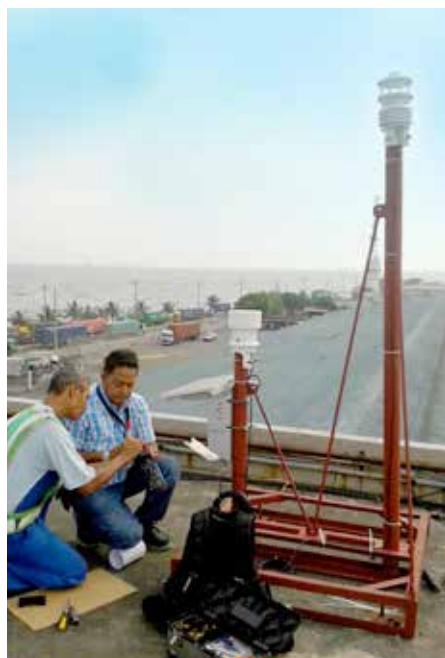
Roll out of automated weather stations — including installation of lightning detectors at selected locations — and training of LGUs and partners continued throughout 2014. WeatherPhilippines's AWS network has now reached 750 meteorological sites nationwide.
