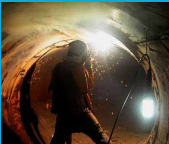
A welder meticulously checks the inside of the 2-km conveyance line of Hedcor's Ampohaw plant for damages during shutdown. The annual rehabilitation of Hedcor's power plants assures that systems can run at optimum performance throughout the rainy season.
