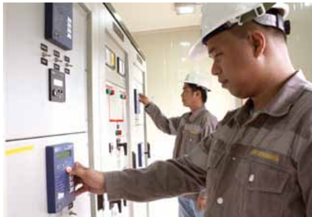
(From left) Engrs. Galen Alovera and Mark Acosta conduct final calibration of the control equipment. These sensitive equipment are now housed in a separate enclosed building to protect it from wear and tear due to harsh weather conditions.
