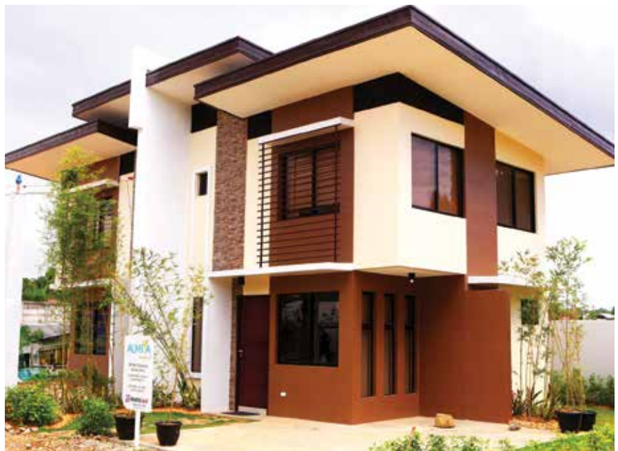
SUN-POWERED. AboitizLand's Almiya is making an effort to reduce the electricity bills of vecinos through the installation of solar panels at the development's units.
