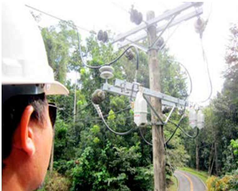
NO MORE POWER OUTAGES. SEZ has installed Cutout-Mounted Reclosers in order to reduce momentary interruptions and permanent outages along the affected line.
