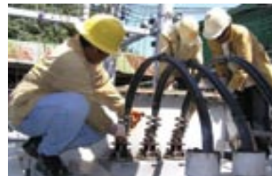
TEAMWORK. Cotabato Light personnel and Transpower crew work as a team to improve back-up power through Preventive Maintenance Servicing (PMS) of generating power transformers.
