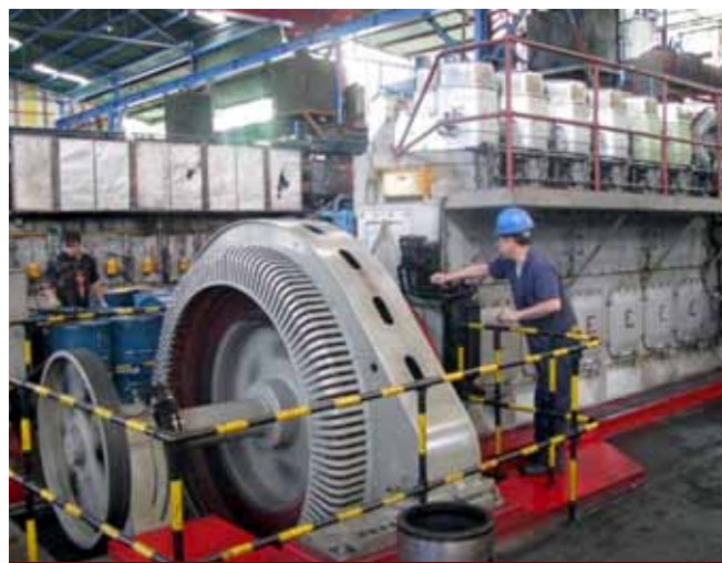
VINTAGE ENGINE BACK ON TRACK. Cotabato Light's 54-year-old Unit-10 (U-10) engine has been restored and is back on track with a maximum load allowable to deliver power to the utility's customers. The U-10 engine increased Cotabato Light's power plant capability to 8.1 MW from 7.45 MW, a performance that is good enough for a vintage engine. The unit had not been operating for more than a year because of three cracked engine cylinder heads, which have been replaced. The US-made Enterprise Diesel Engine was manufactured in 1956 and bought second hand from Jolo, Sulu and commissioned at Cotabato Light in 1967. (Jonathan P. Acosta)
