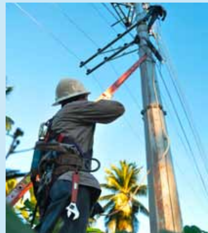
GEARING UP. Powerline technicians open the transmission line from Sibulan Hydropower Plant 1 to Puan Substation in preparation for the testing of the two power generating units of Plant 1. The plant is set to deliver 92 GWh hours of clean energy annually to Davao City electric consumers soon through the Puan Substation. Plant 2 of Sibulan Hydropower Project started supplying energy to Davao City in April this year. (Karen Padawag)
