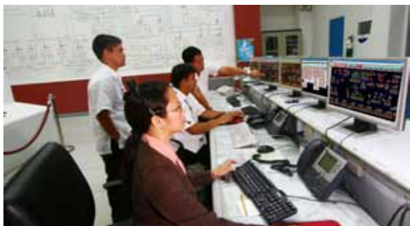
Systems Operations manager Ledio Peñafiel instructs his staff on the Supervisory Control and Data Acquisition (SCADA) system as supervisor Roger Alinsub observes. The SCADA allows engineers to remotely control switches in the substations and along the distribution lines. The interconnection of the company facilities using fiber optics allows the use of the SCADA.
