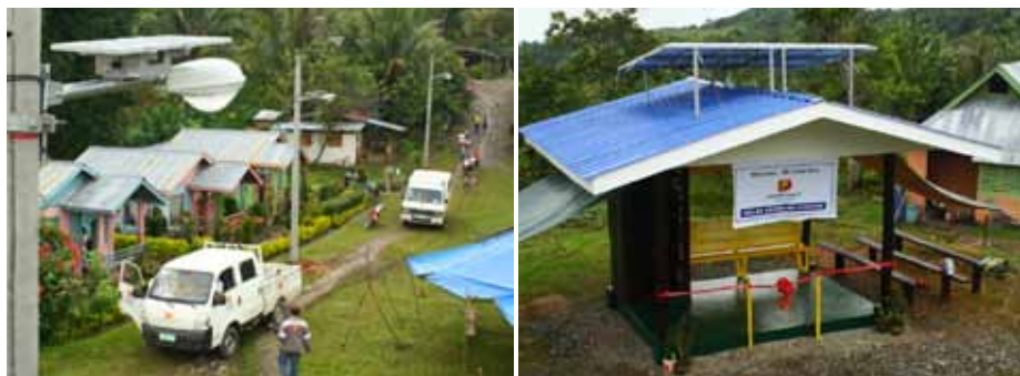
(Above) Solar-powered streetlights illuminate the center ground of the GK Violet Hills Village in Kibalang, Marilog. The solar panels (right) installed above the charging station at GK-Violet Hills in Kibalang, Marilog collect the energy from the sunlight and store it for use in charging the batteries assigned to each housing beneficiary.
