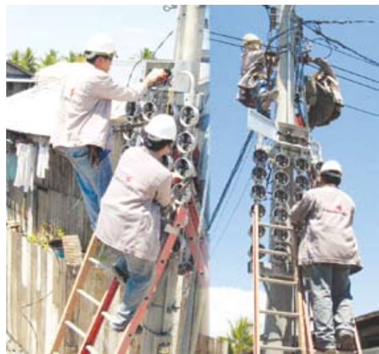
Cotabato Light engineers and linemen work side-by-side in assembling, installing, and energizing the 24-meters-in-one MOP multi-clusters at Bulyao, SK Pendatun Ext., Cotabato City.
